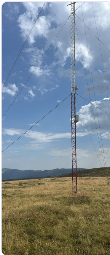
A radio mast on the network's rural backbone.
